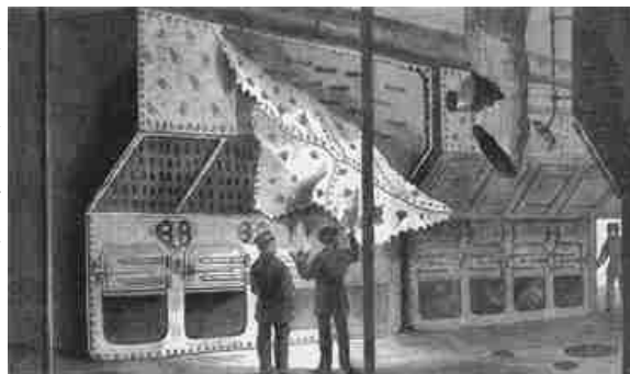
HMS Thunderer's Boilers
